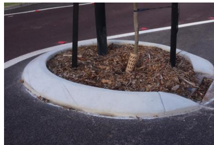
Fig 3 – Close-up of a City of Bayswater pinch point
