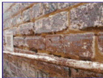
Deteriorating mortar noted.
