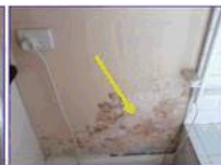
Past moisture damage noted.
