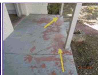
Concrete cracking noted.
