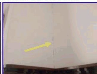
Cosmetic cracking noted
