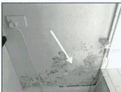
Past moisture damage noted.
