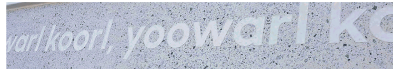
Material: Etched text into exposed aggregate.
