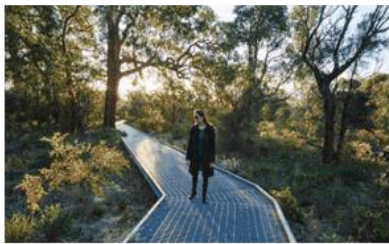
Figure 55. Raised perforated steel boardwalk.
