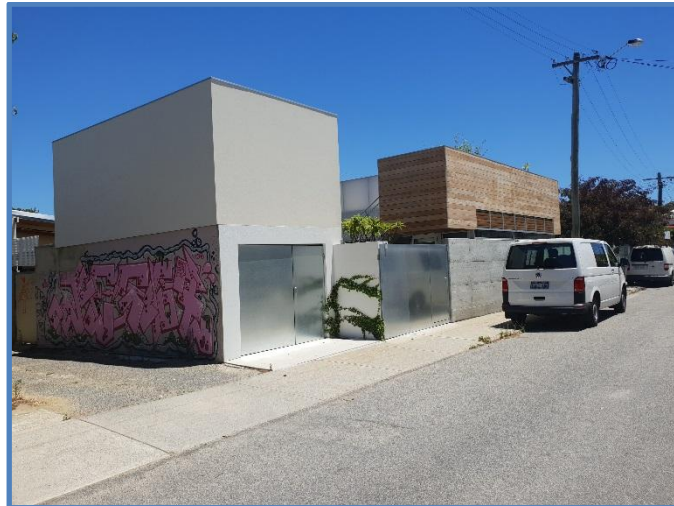
Structure at 16 Orange Avenue, fronting Hope Street
