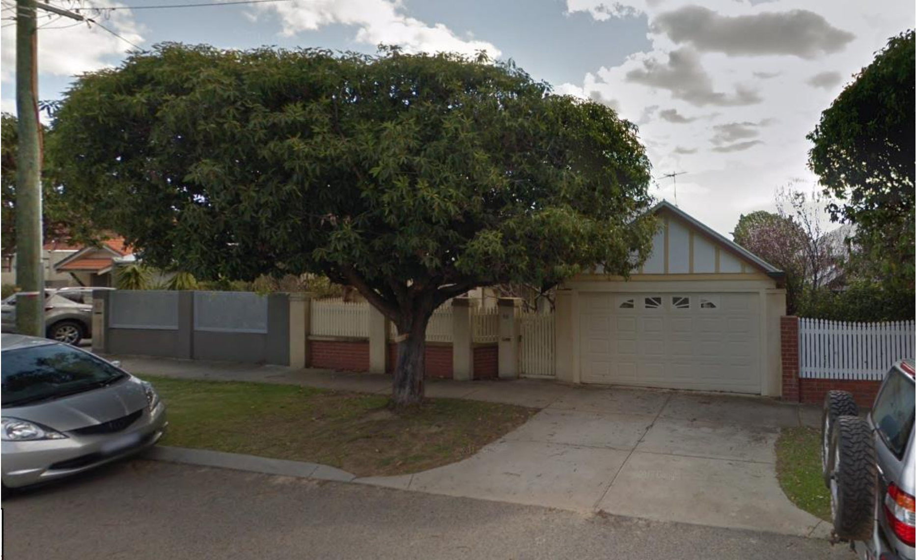
69 Kalgoorlie Street Mount Hawthorn
