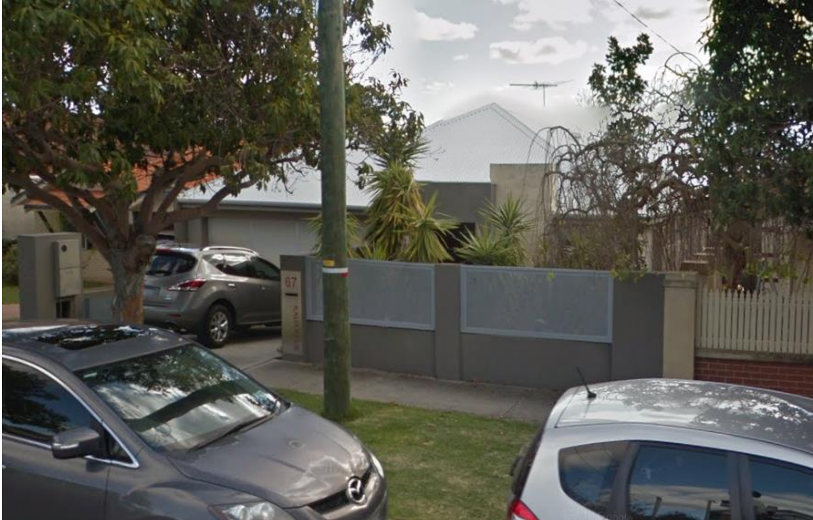
67 Kalgoorlie Street Mount Hawthorn
