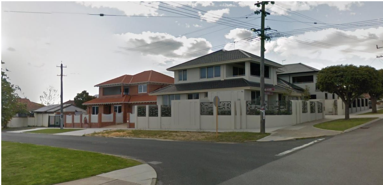
32 Ashby Street and 55 Kalgoorlie Street Mount Hawthorn.
