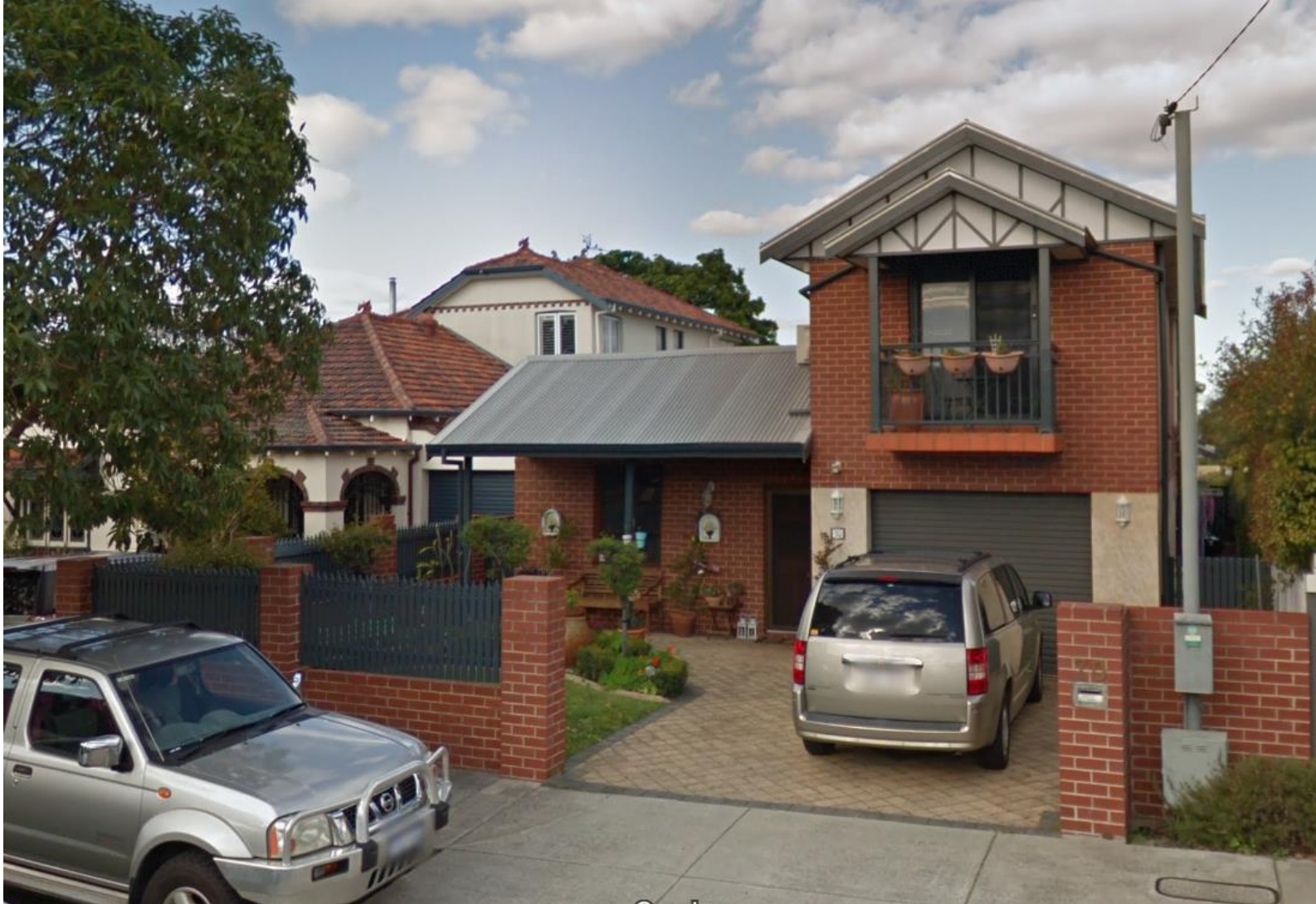
70 Kalgoorlie Street Mount Hawthorn
