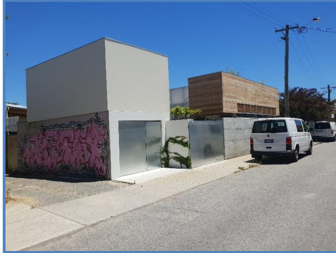
Structure at 16 Orange Avenue, fronting Hope Street
