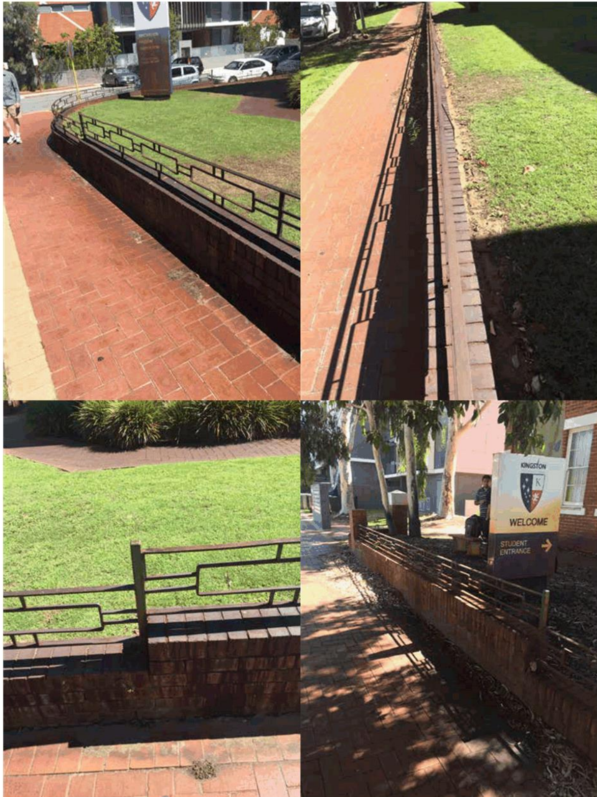
Photos showing current condition of brickwork & wrought iron fence heavy iron staining and rusting of iron is evident
