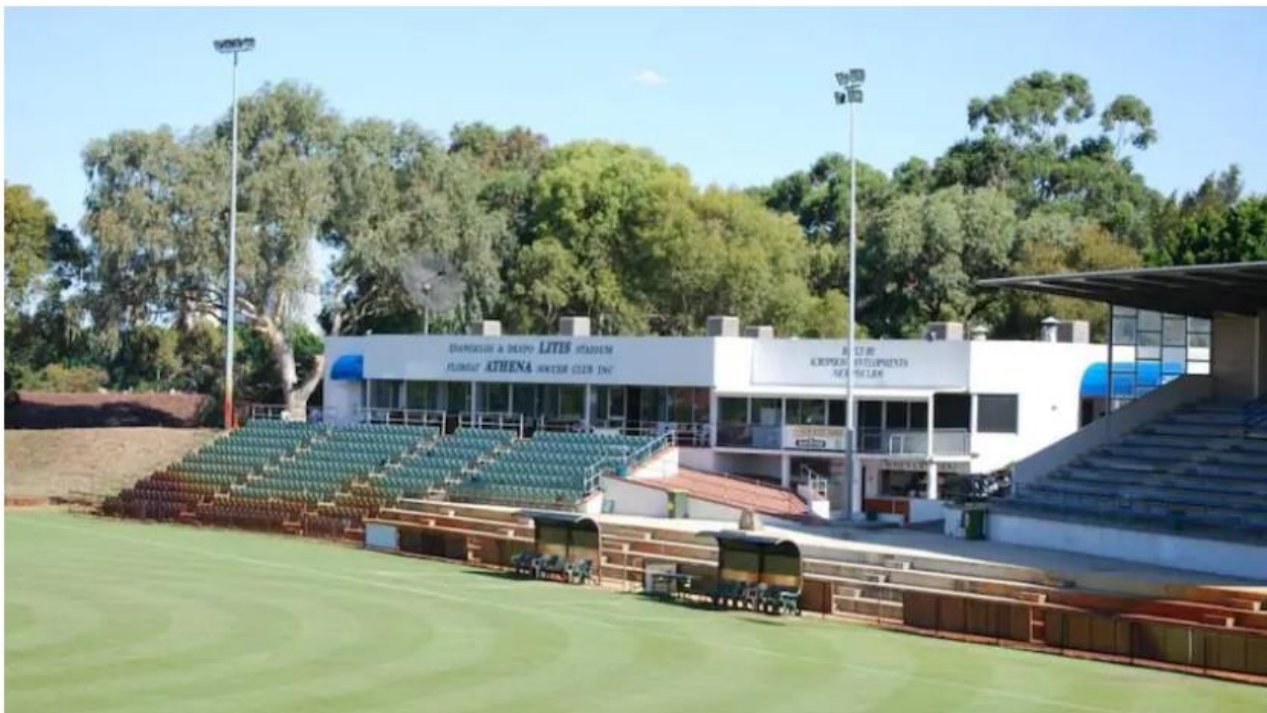
Figure 1 – FAFC’s Current Facilities
