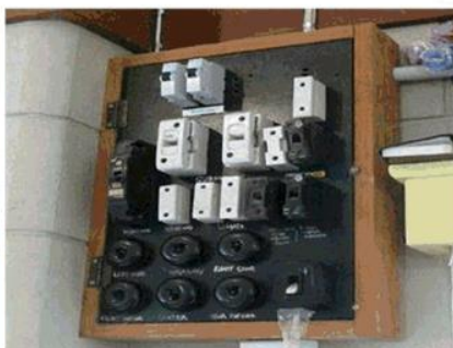
Electrical Switchboard and ceramic fuses
