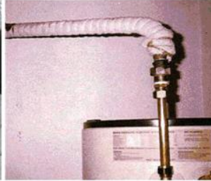
Coolgardie Safe insulation lagging
