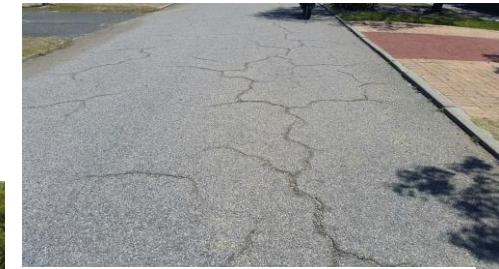
An interim crack sealing, or preventative maintenance, to extend the life of the asset (Fleet St – Access Road)
