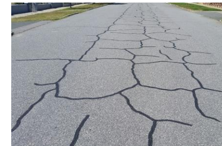
An interim crack sealing, or preventative maintenance, to extend the life of the asset (Fleet St – Access Road)
