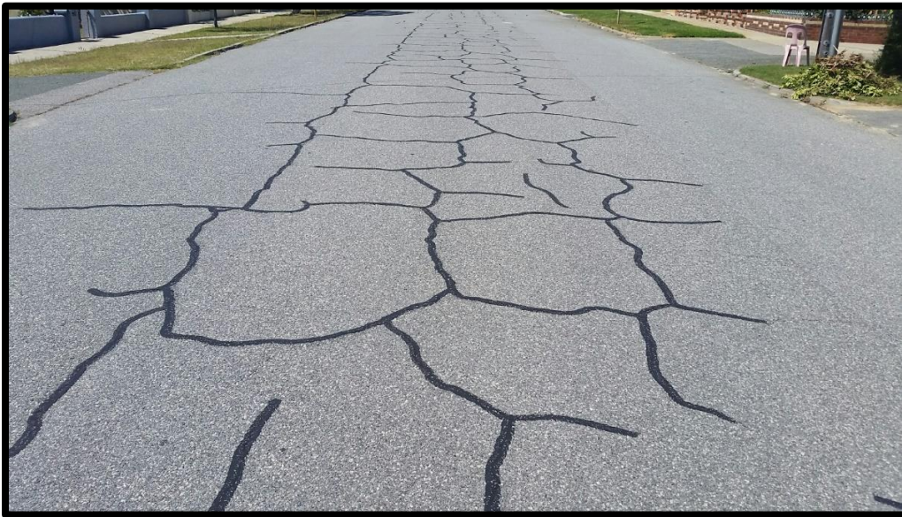
An interim crack sealing, - preventative maintenance, to extend the life of the asset (Fleet St – Access Road)
