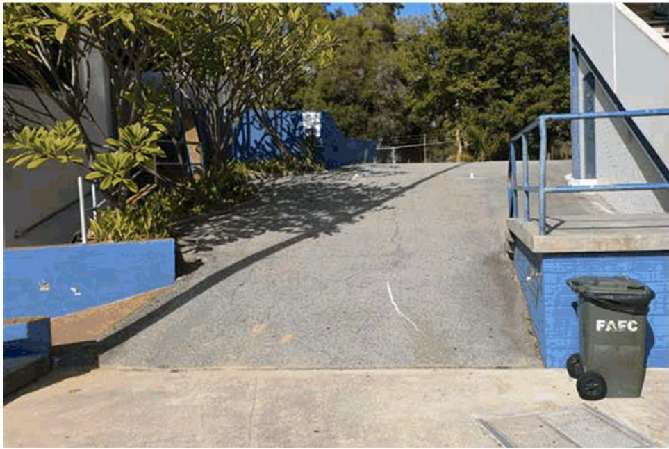
Access grades non-compliant
