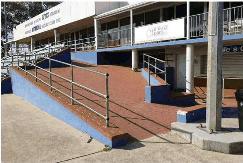
Access grades non-compliant
