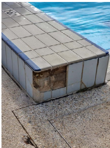
50m pool (bulkhead tiles delaminating)
