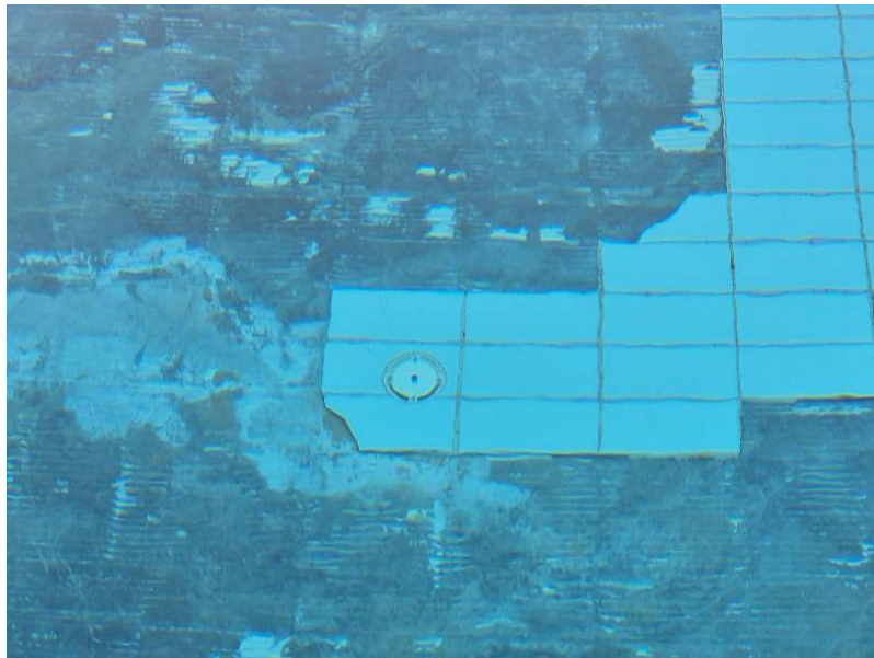
30m pool (close up of tile delamination)
