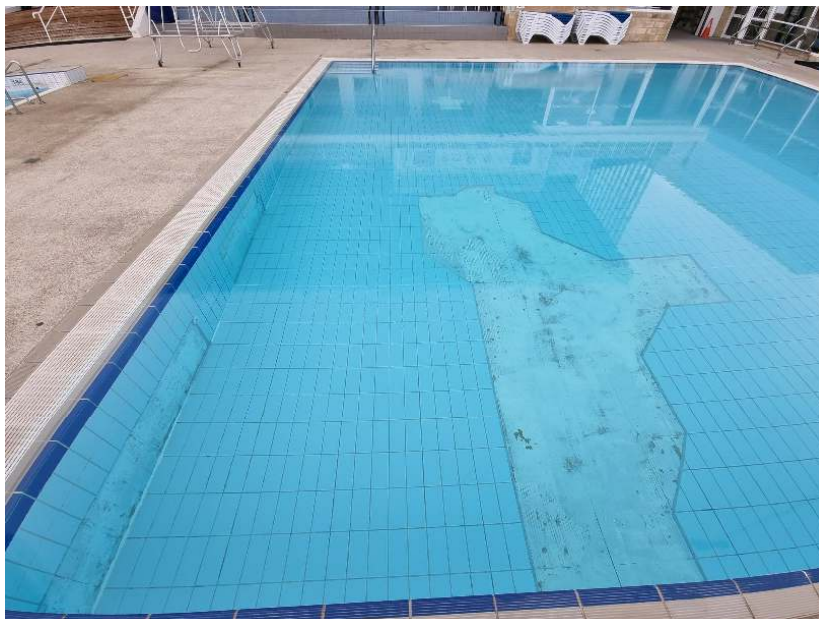
12m pool (tile delamination on floor and wall – edges sealed July 2022)
