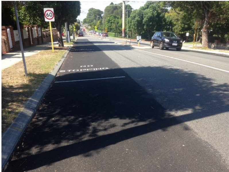
Vincent Street – Full lane resurfaced
