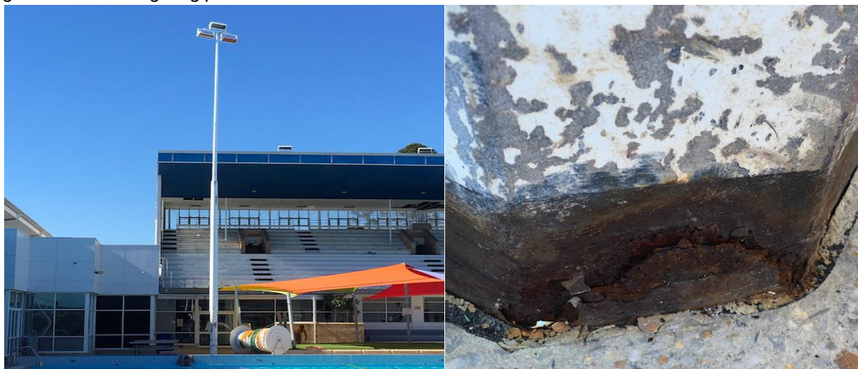
Fig. 3 – Pool deck lighting poles
