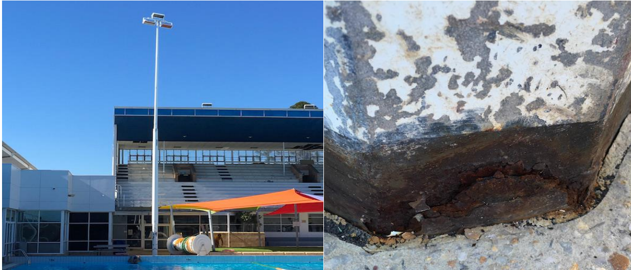
Fig. 3 – Pool deck lighting poles
