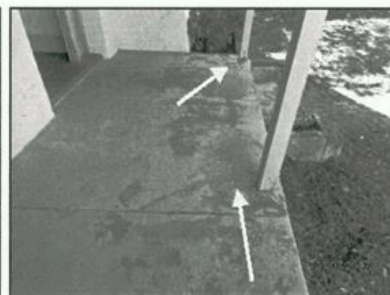
Concrete cracking noted.
