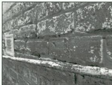
Deteriorating mortar noted.
