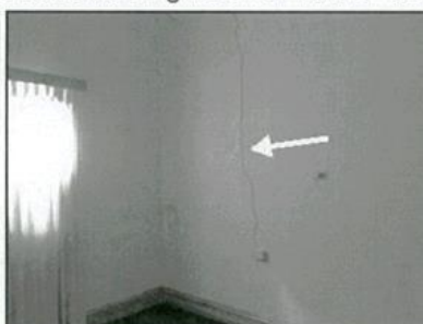
Significant cracking noted.
