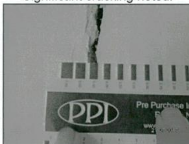
Significant CRACKS in areas.
