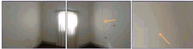
Significant cracking noted.
