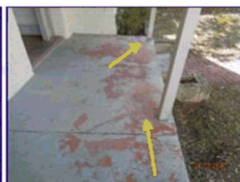
Concrete cracking noted.
