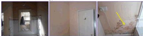
Past moisture damage noted.
