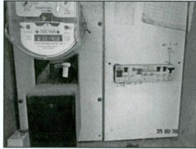
RCD's fitted.
