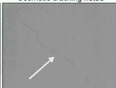
Cosmetic cracking noted
