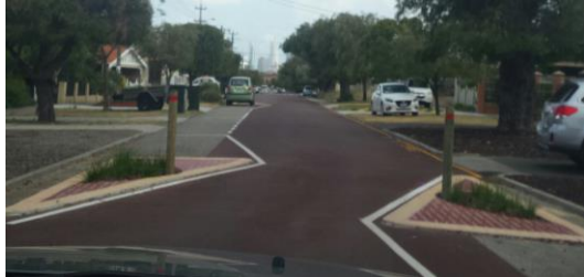
Fig 1 – Typical Shakespeare Street pinch point
