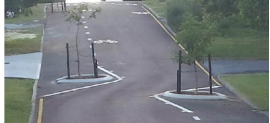
Fig 2 – Typical City of Bayswater pinch point
