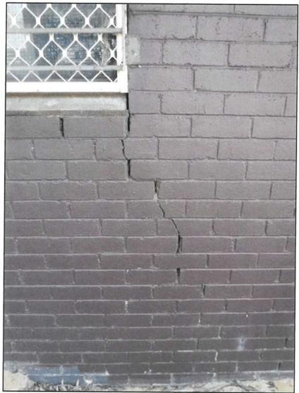
Photograph 2 Cracking on the south facing external wall.
