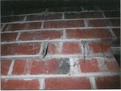
Photograph 3 Cracking on the eastern wall was up to 20mm wide.
