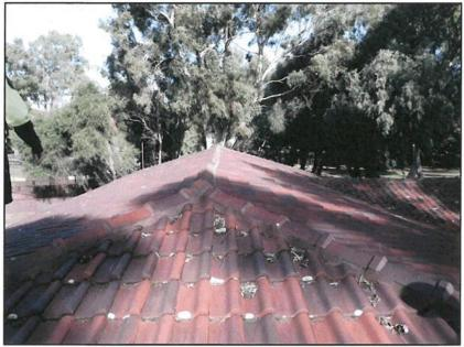
Photograph 7 The ridge of the building is no longer straight.
