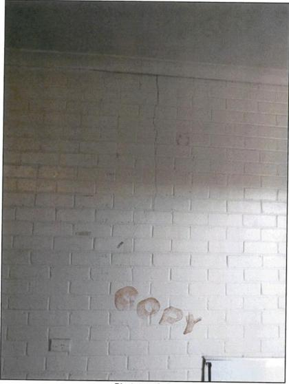
Photograph 4 Vertical cracking in the western section of the building.
