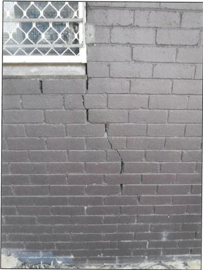
Photograph 2 Cracking on the south facing external wall.
