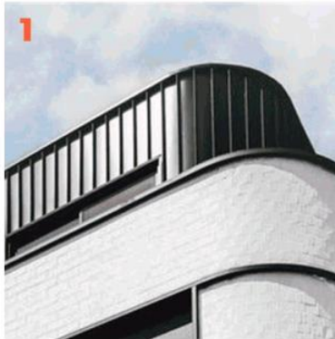
1. Lightweight upper floor cladding to contrast with masonry materials at lower levels.
