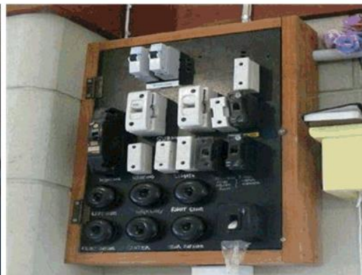
Electrical Switchboard and ceramic fuses
