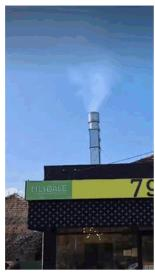
Figure 12: Vertical rise of the plume under no to very light wind
