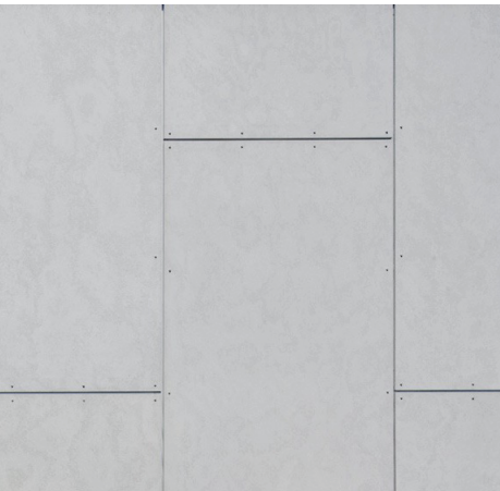
FC-01 Fibre cement cladding - Type 1 Colour: Grey Location: External walls (north and west)
