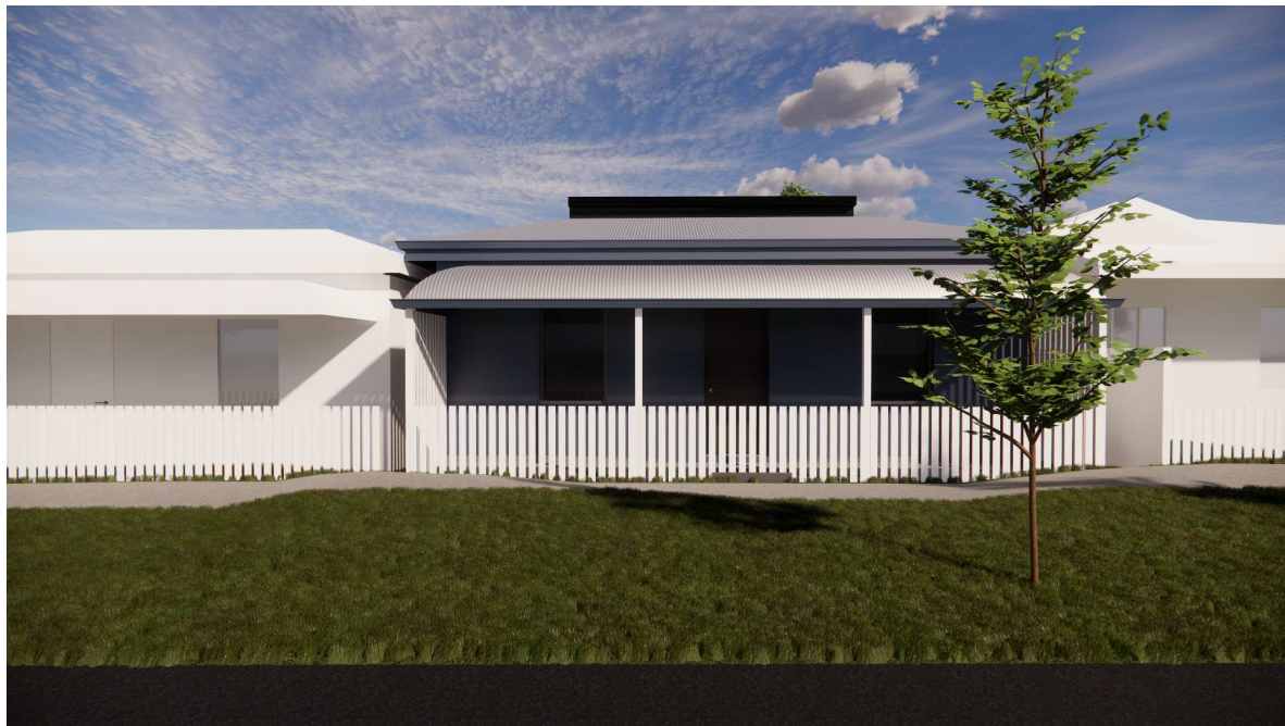
LINCOLN ST VIEW 1 South - Road at eye level
