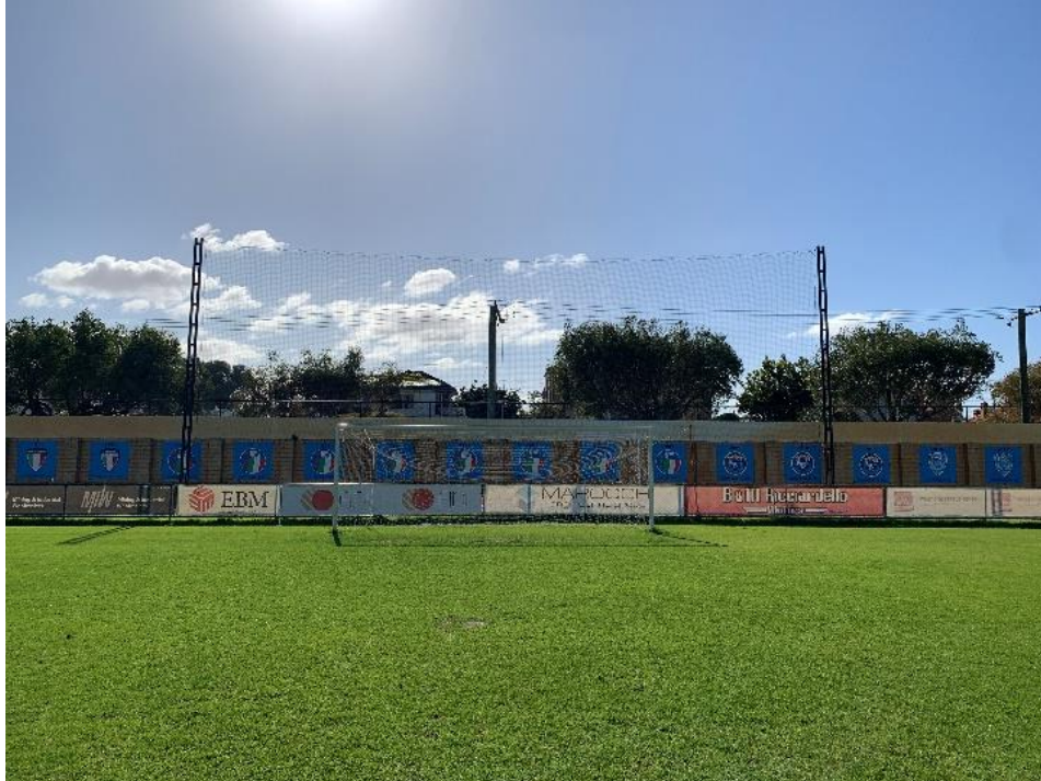
Figure 1 – View of the Soccer Net Structure from Perth Soccer Club (Looking North).
