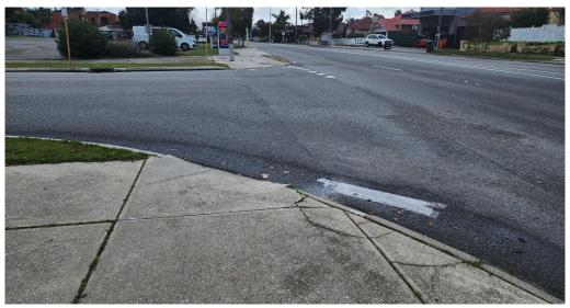
Photo 15: Crossing at end of Ellesmere St does not align correctly and has poor pedestrian ramps.
