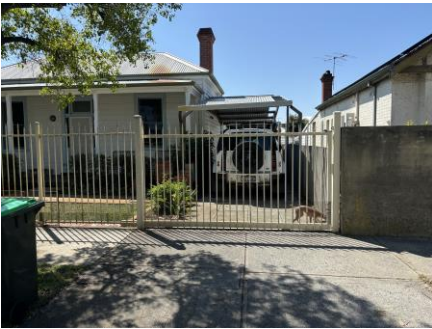
Fig.2: Here is a side view of the location clearly showing ample room for 2 cars in the driveway behind the closed gate within the property boundary
