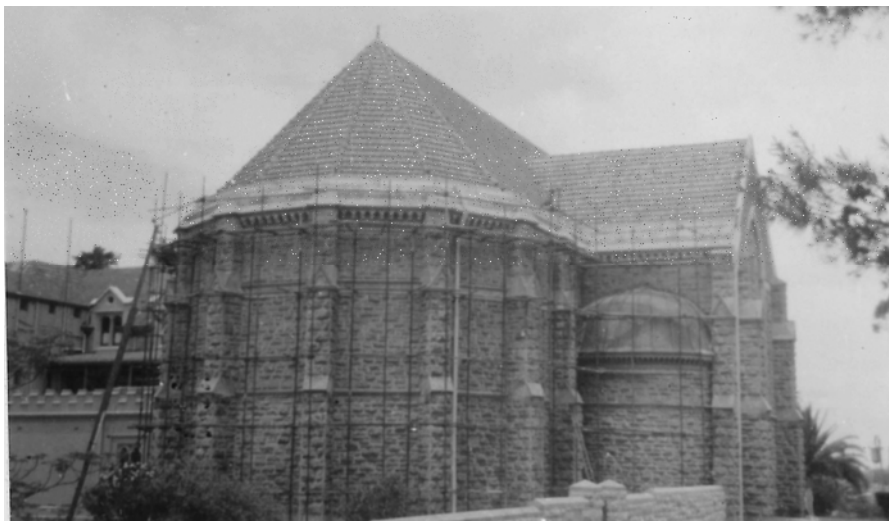
Photograph 35 Scaffolding round the Apse during guttering repairs, November 1956. These works may have included fitting a gutter mounted upon the parapet wall – the system which is extant today. Photograph held by Redemptorist Fathers.
