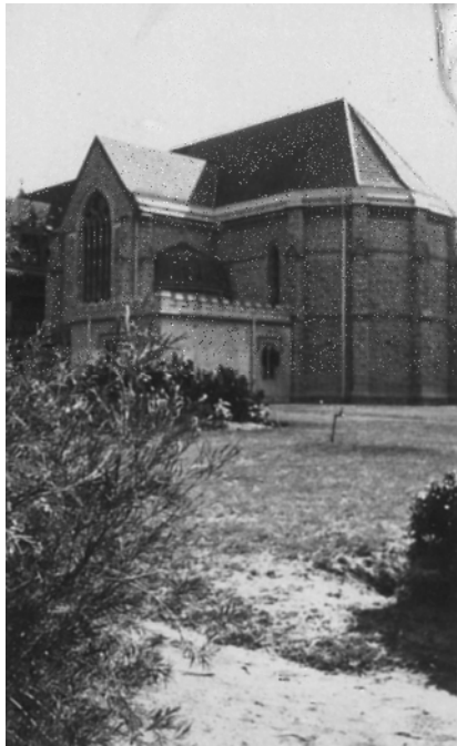
Photograph 12 Showing the 1922 extension to the church, c.1956. Note that the parapet to the top of the sanctuary and transepts was not crenellated as suggested in the design drawings. This photograph was taken after re-roofing and shows that roof details have been removed, including gablets, and dragon back ridge tiles. Photograph held by Redemptorist Fathers.
