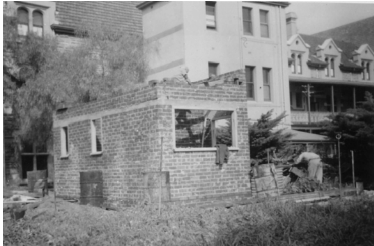
Photograph 31 Storehouse under construction 1955. Note the banding to the north elevation of the 1912 northern extension has been painted over. Louvres had not yet been fitted to the upper floor windows on the eastern extension. Photograph held by Redemptorist Fathers.
