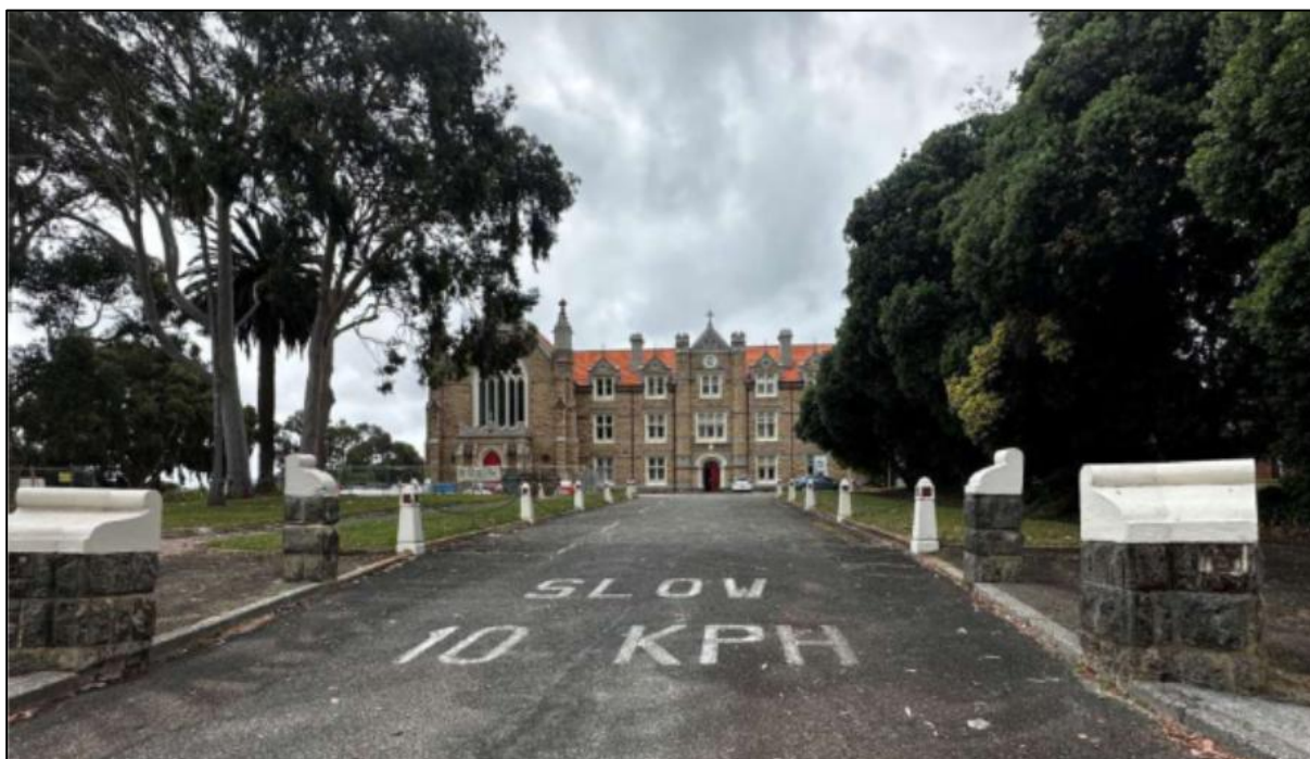
Figure 3: Existing landscaping shown at the Vincent Street main entrance, with all New Zealand Christmas Trees to the right proposed to be removed.
